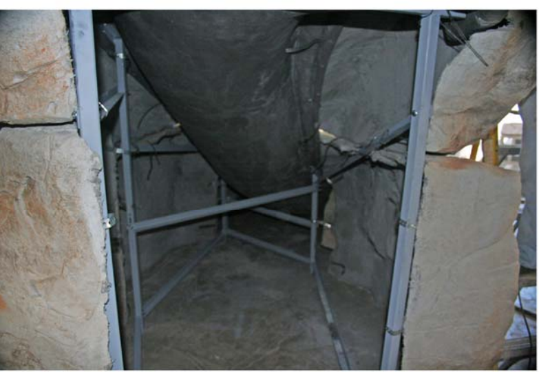
3. Secure cast pieces to steel frame
