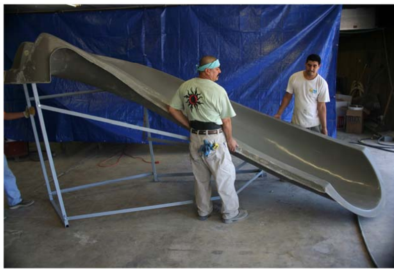
2. Set slide and bolt to steel frame
