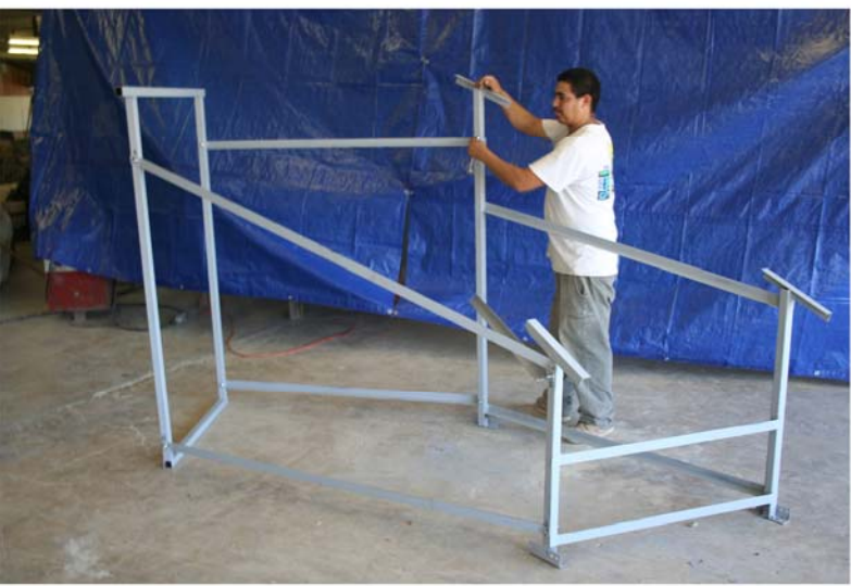
Installation: 1. Bolt steel frame pieces and secure to concrete pad.
