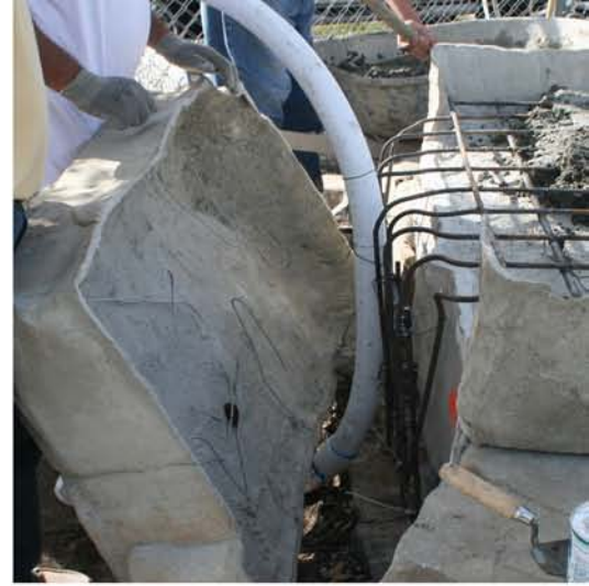
Extend 2 inch pvc plumbing before setting back casting #5. Also run sleeves for lighting.
