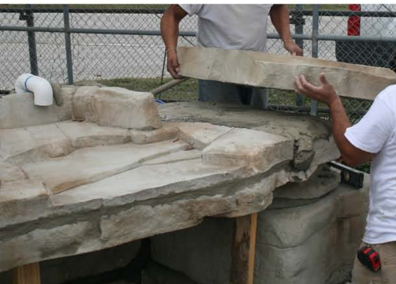
Add 2 inches of concrete fill on each side of grotto top and mortar in top rocks #8 and #9. Add two 90's to 2inch return line to discharge onto grotto top. Set cap rock #10 to hide pipe.
