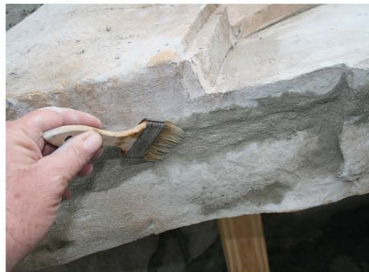
Finish seam between grotto bottom and top. Add accent colors to waterfall pieces. Set small rocks as desired or to divert waterflow.
