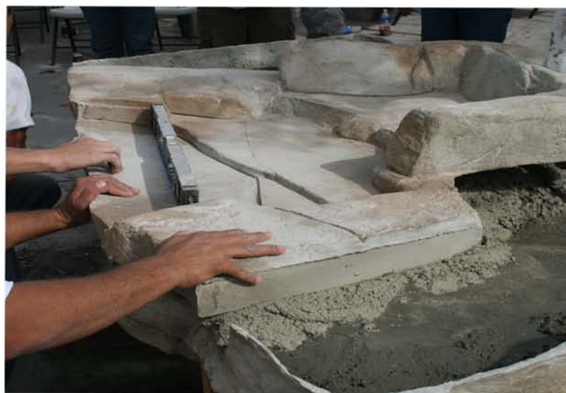
Set grotto top piece #7 in fresh concrete or mortar. It must be level and shape should match the grotto bottom piece. It will drain down when pump is off if set properly.
