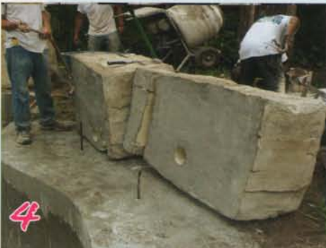
4 Dowels in place, ready to mortar pieces.
