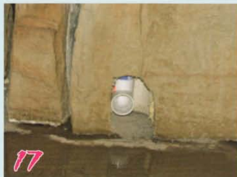
17 Connect plumbing at back of base piece. Hide pipe with extra rocks provided in kit.
