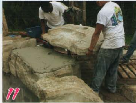
11 Set lower shelf piece with mortar; match up pipe columns.
