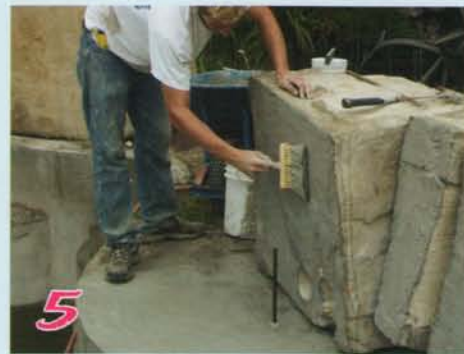
5 Bonding is critical. RicoRock Waterproofing can be brushed on cast pieces.
