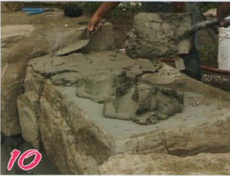
10 One inch mortar bed for next layer of castings.
