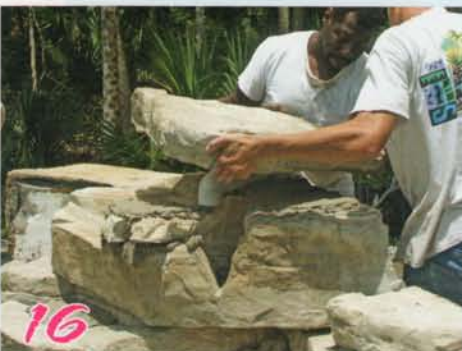
16 Mortar cap rocks or use epoxy for less mortar clean-up. Rake joints about 1/2 inch.
