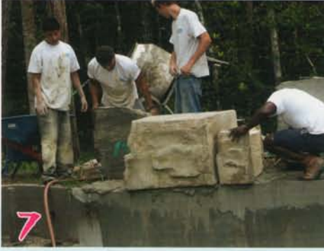
7 Set base pieces to overhang pool 1-2 inches. For off-set see Installation Notes.
