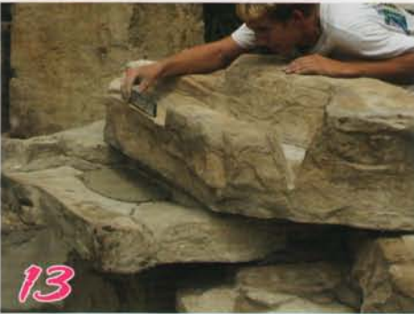
13 Set Basin Piece, match pipe columns.
