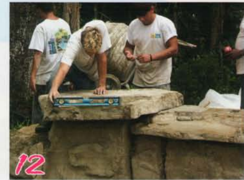
12 Set upper shelf piece; must be level from right to left but not from front to back.
