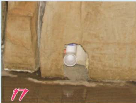
17 Connect plumbing at back of base piece. Hide pipe with extra long piece (cut to fit).
