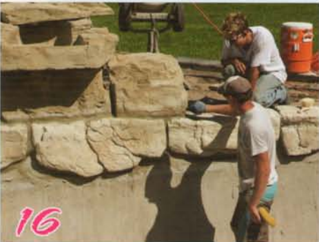
16 Mortar cap rocks. Clean excess mortar & rake joints about 1/2 inch.
