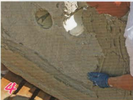
4 Scrub a thin layer of mortar on the bottom of base pieces for better bonding.
