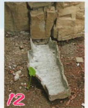
12 Use the long extra piece (Cut to Fit) for a gap in back if needed.
