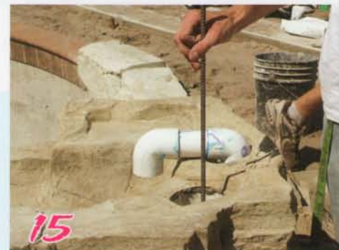
15 Add rebar piece & finish concrete column to top of basin piece.
