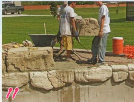
11 Set other side boulder. On a radius. There will be a gap in the backside.
