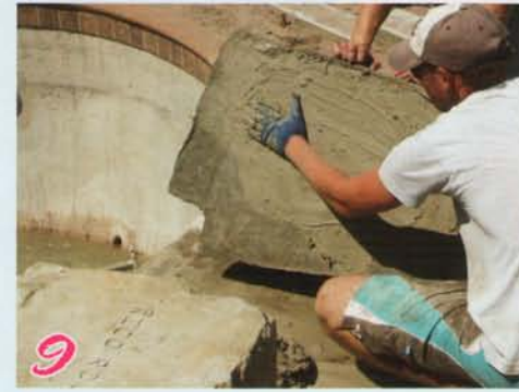
9 Wet & butter up side boulder with mortar.
