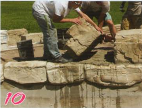
10 Set side boulder & mortar gap with base piece.
