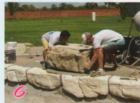
6 Set base over rebar dowel and press into mortar bed.
