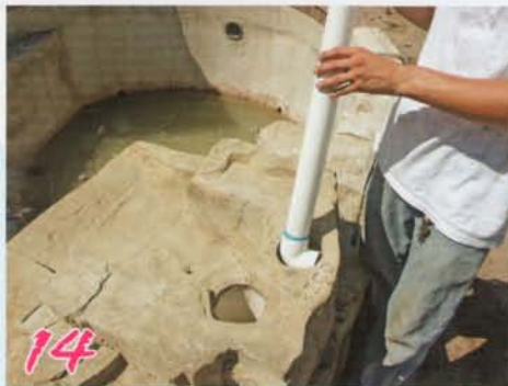
14 Drop plumbing sleeve in hole. Tighten threaded plug if you plan to pressure test line.
