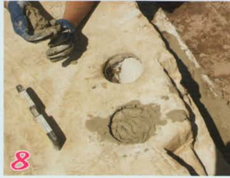
8 Fill concrete column with concrete.
