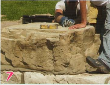
7 Base piece should be level side to side but not necessarily from front to back.
