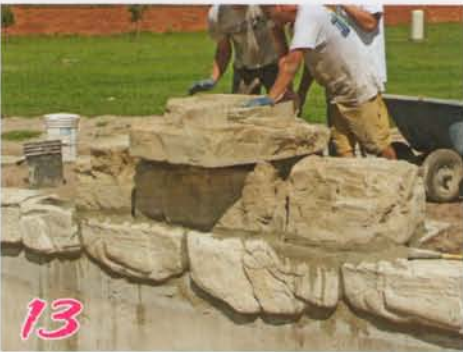
13 Set basin on 3/4" mortar bed. Level from left to right. Match up plumbing & concrete holes.
